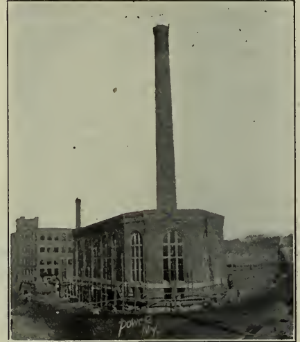
FIG. 1. THE NEW STARRETT POWER HOUSE
